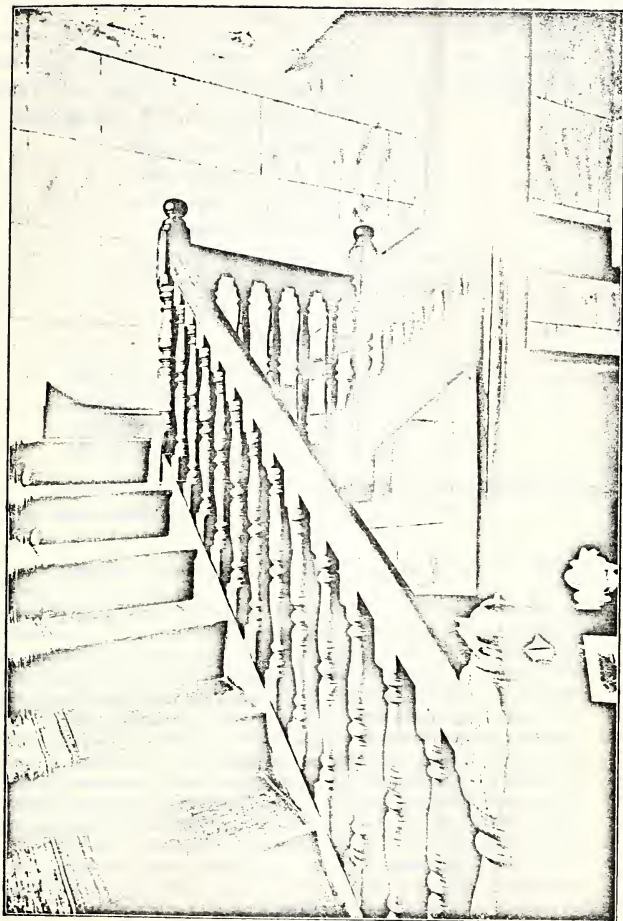
STAIRCASE AT GARSDON MANOR HOUSE.
