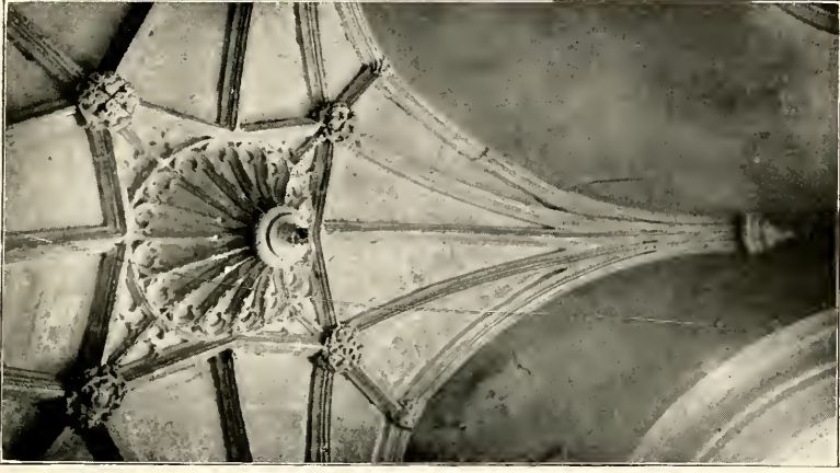
CEILING OF NORTH PORCH, [facing p. 160.
