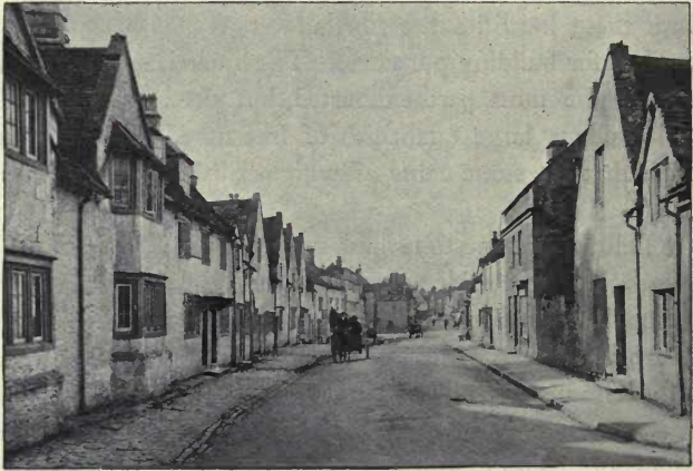
Flemish Houses, Corsham
