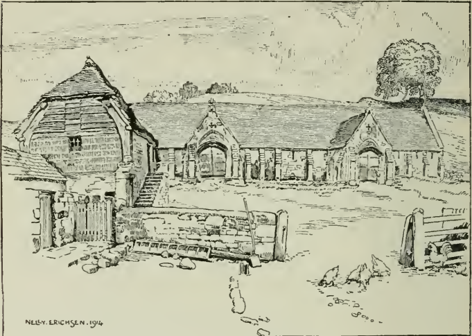
The Barton Barn, Bradford-on-Avon.
