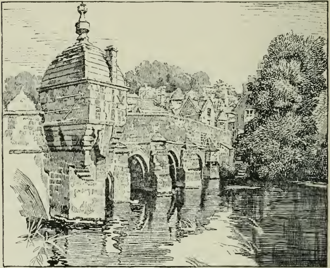
Bridge Chapel, Bradford-on-Avon.
