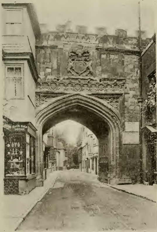
HIGH STREET GATE, NORTH FRONT, SALISBURY
