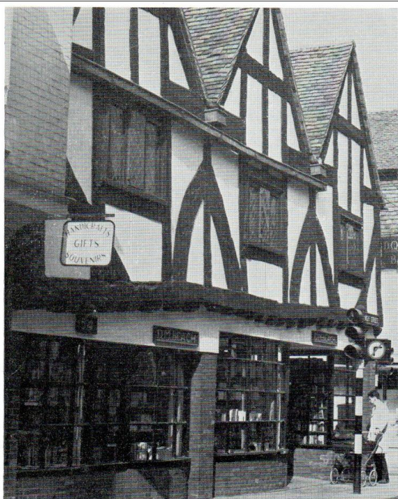
• Above : Beach's Book Shop at Salisbury showing the warped woodwork.
