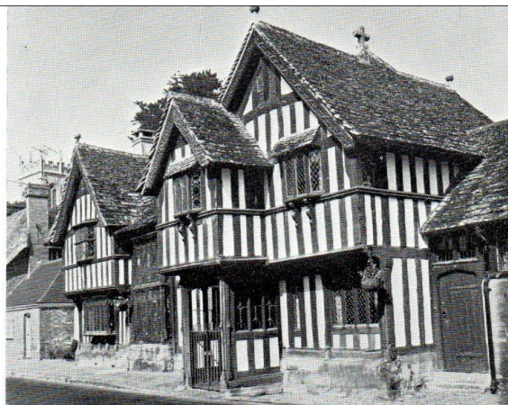
● Above : Porch House at Potterne, one of the best examples of its kind in England.
