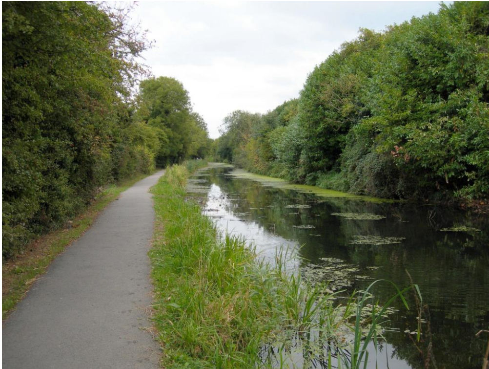
A Wiltshire Stretch of the Wilts & Berks Canal
