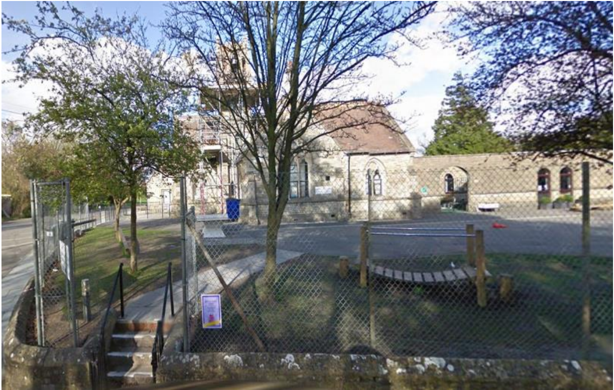
View of Sutton Veny School opposite the Milestone
