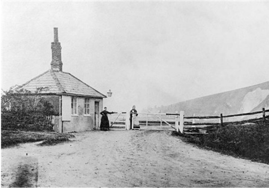
A Typical Toll Gate and House of the late 1800s
