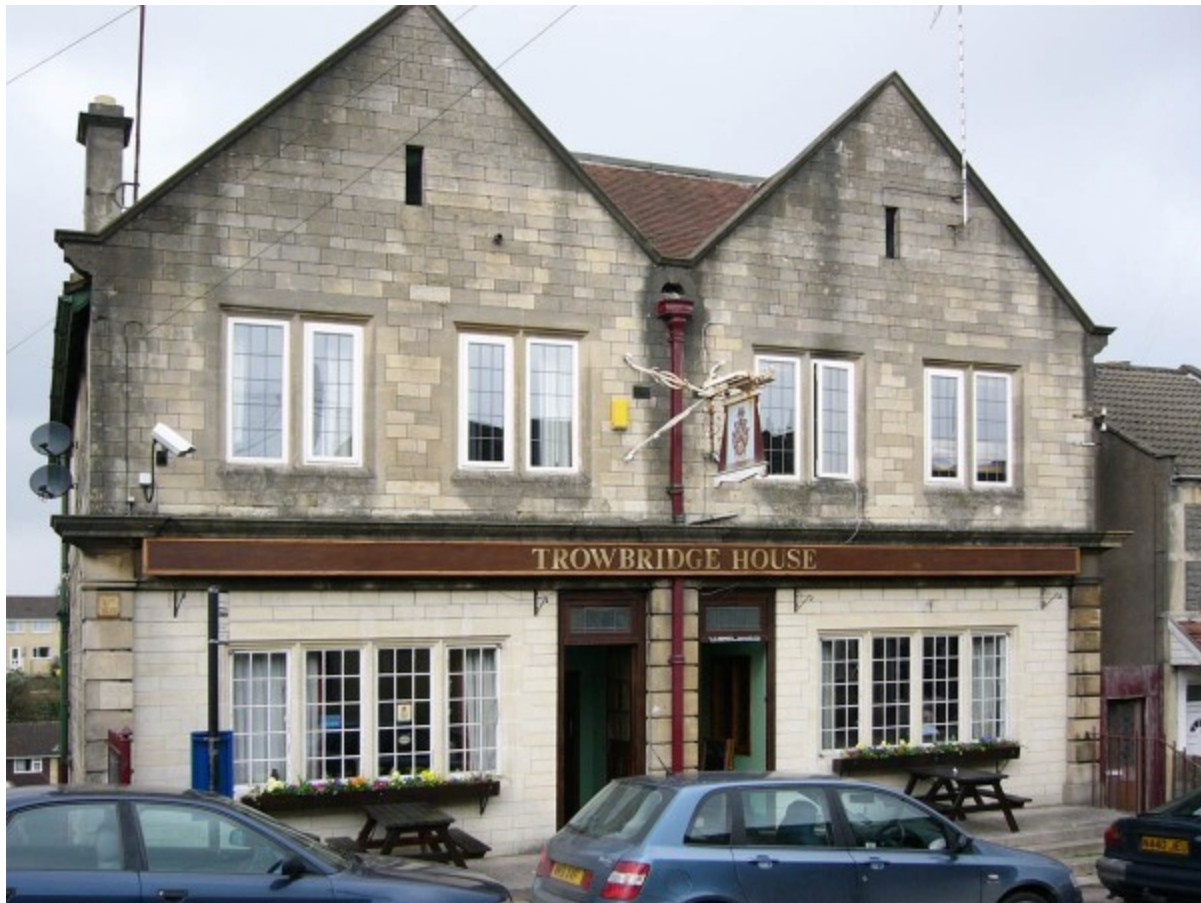
The Former Coronation House, Bath built by Ushers Brewery as an Off-License in 1923
