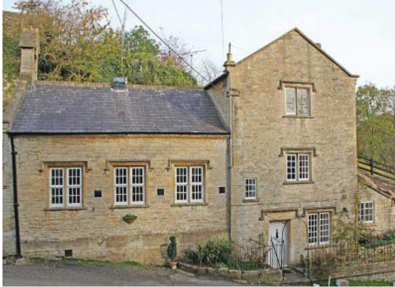
North Wraxall School courtesy of Wiltshire & Swindon History Centre
