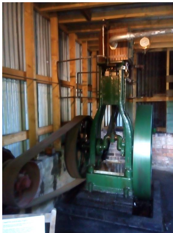
Winding machinery for the pit shaft cages.
