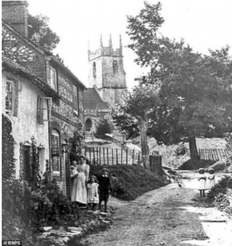
Abandoned: The village, pictured around 1900, was commandeered by the army so soldiers could practice ahead of the D-Day landings during WWII
