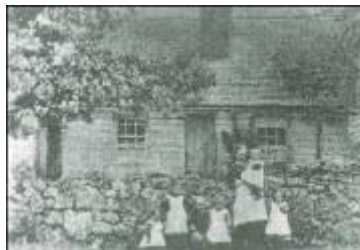
A Fencible cottage - the Fencibles built these themselves.
