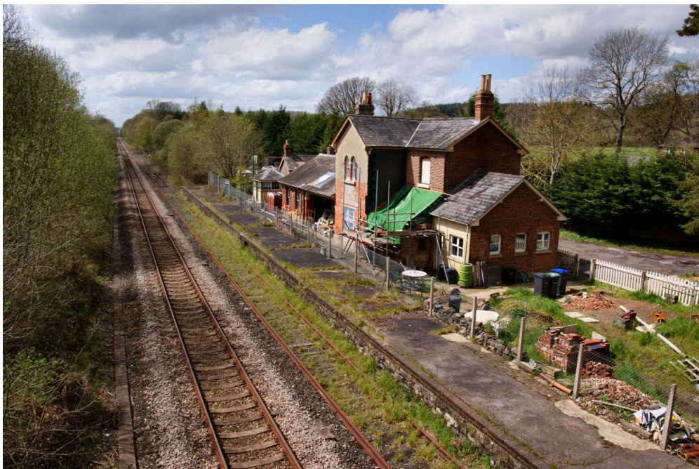
Dinton Railway Station – taken May 2012 by Andrew Stacey
