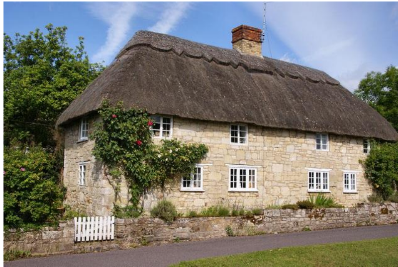
Parkside Cottages (Photo by Andrew Stacey 2011)
